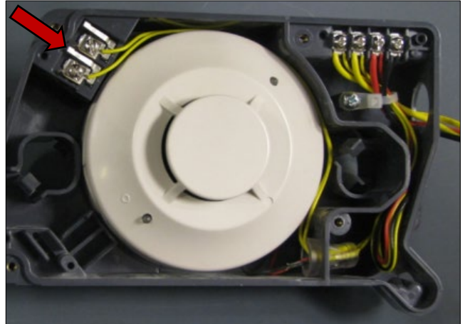
Tamper Switch Location
